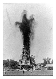
At the beginning of oil exploitation, one just have to drill a well and oil will gush from the underground as in the picture of an American oilfield. However, this easy part does not last very long and secondary and tertiary techniques have to be used in order to recover the most of the oil. In this exercise we will try to understand the mechanisms of oil recovery and the different issues associated.
